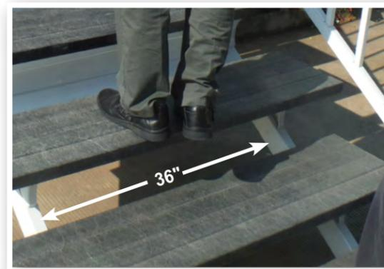
QuickStep stair treads shown with QuickStep stair stringers at 36" centers.
