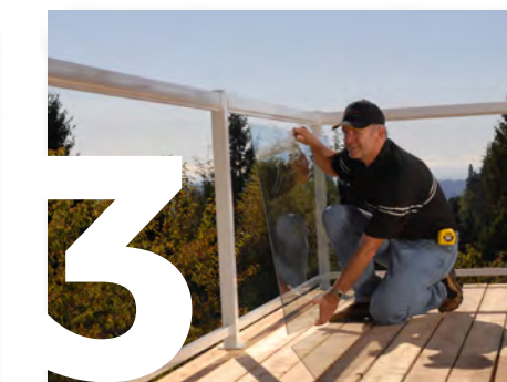
INSTALL PICKETS OR TEMPERED GLASS PANELS
