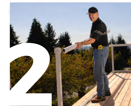
INSTALL TOP & BOTTOM RAILS
