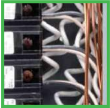
Pigtail Neutral Connections
