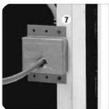
The bracket mounts directly onto the stud.
