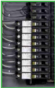
Plug-on Neutral Connections
