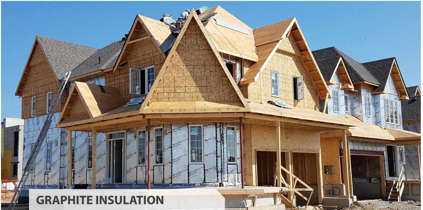
SilverBoard Graphite XS is a high performance, non-structural, rigid insulation board made from Expanded Polystyrene (EPS) with a layer of reflective metalized polypropylene film lamination on both sides.
