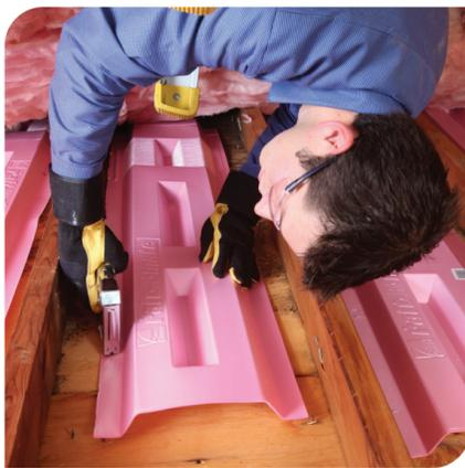
To calculate the number of attic rafter vents required, please consult applicable building codes for required ventilation area.
