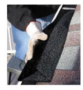
5. Do not stretch the material to make it fit as it will shrink back to its original form and leave gaps.
