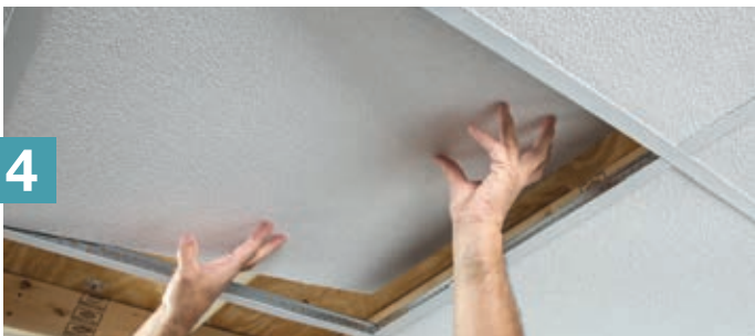
Install ceiling panels
