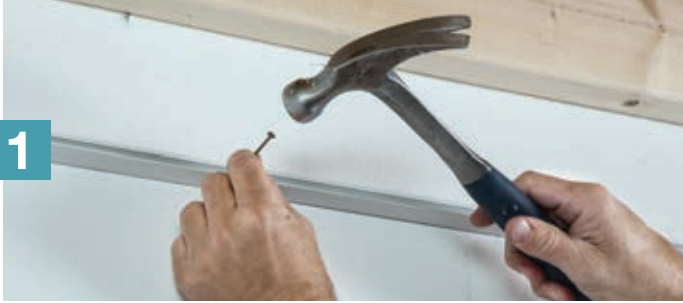
Install wall molding
