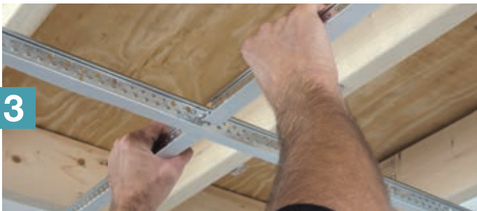
Install cross tees
