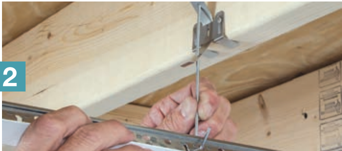
Suspend main beams with hanger wire or NEW QuickHang™ hardware* (shown above: QuickHang hooks and brackets)
